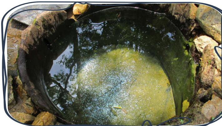
**Panam Keni** - A native to Wayanad district of Kerala, panam kenis are special wells. Made by soaking the stems of toddy palms in water for a long time so that the core rots away until only the hard outer layer remains. These cylinders are then immersed in groundwater springs in fields and forests. A source of abundant water even in the hottest summer months.
