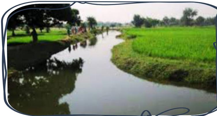
**Ahar Pynes** - Indigenous to south Bihar, this irrigation system leverages the natural marked slope of the terrain. It is embanked on the remaining three sides. Pynes are diversion channels made to utilise river water in agricultural fields. Starting out from the river, they run through fields to end up in an ahar.
