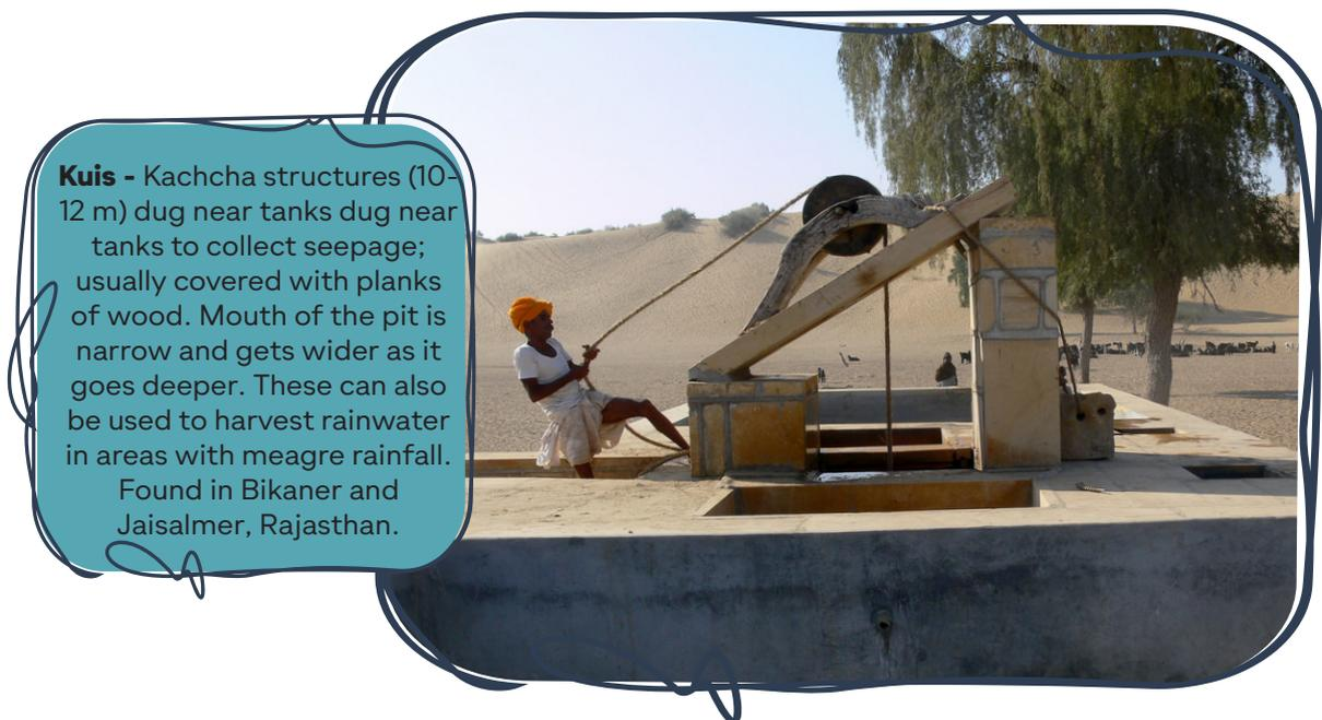
**Kuis** - Kachcha structures (10-12 m) dug near tanks dug near tanks to collect seepage; usually covered with planks of wood. Mouth of the pit is narrow and gets wider as it goes deeper. These can also be used to harvest rainwater in areas with meagre rainfall. Found in Bikaner and Jaisalmer, Rajasthan.
